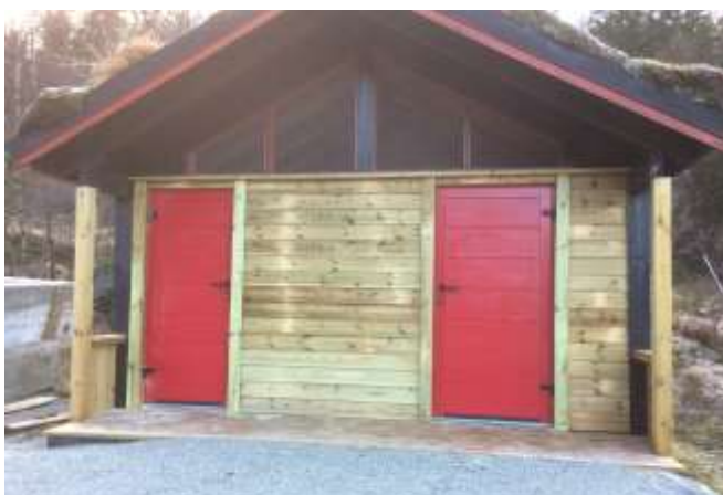
Reparert toalett i Brekko, universell tilrettelegging
